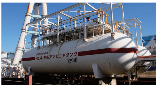
Ammonia storage tanks for denitrification
