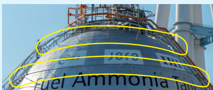
Sprinkler system for the ammonia fuel tank (highlighted in yellow)
